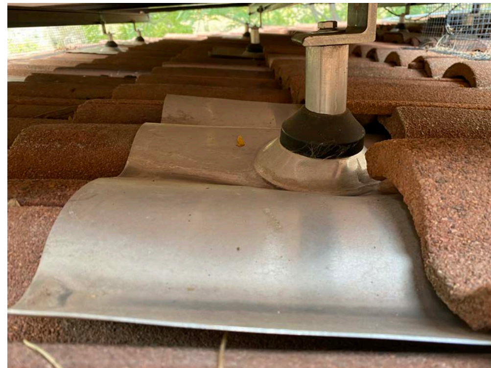
Flashing for tile roof
