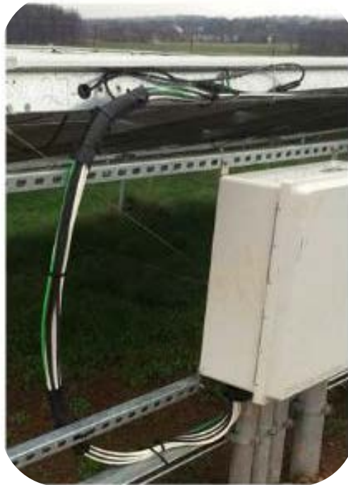
Wire ties to rack
