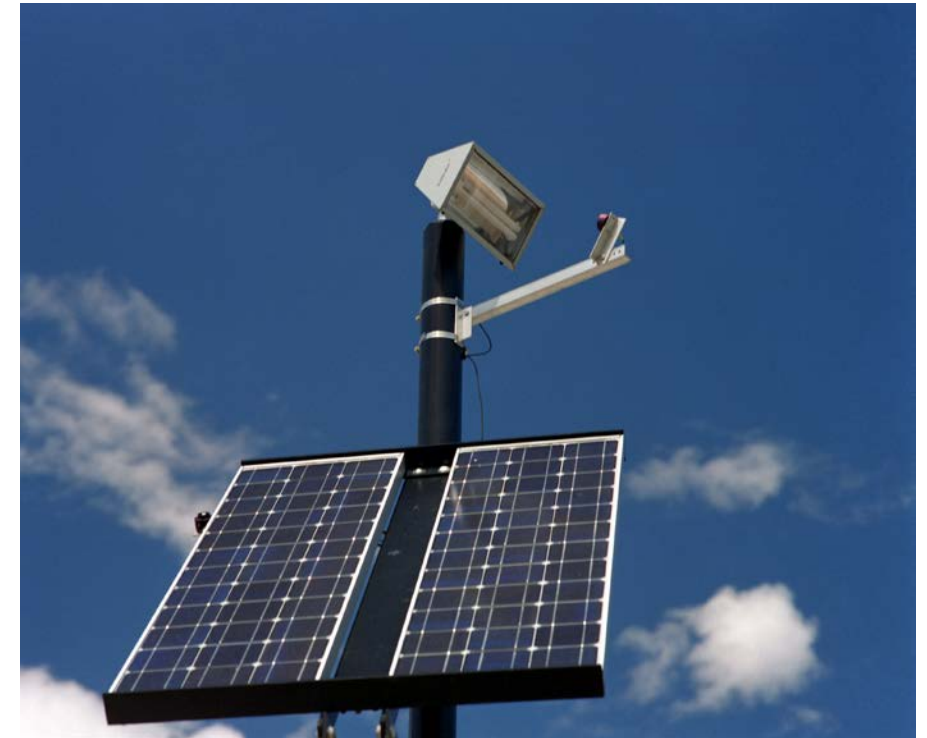
Photovoltaic-powered light in Golden, Colorado. Image by Warren Gretz / NREL 01654
