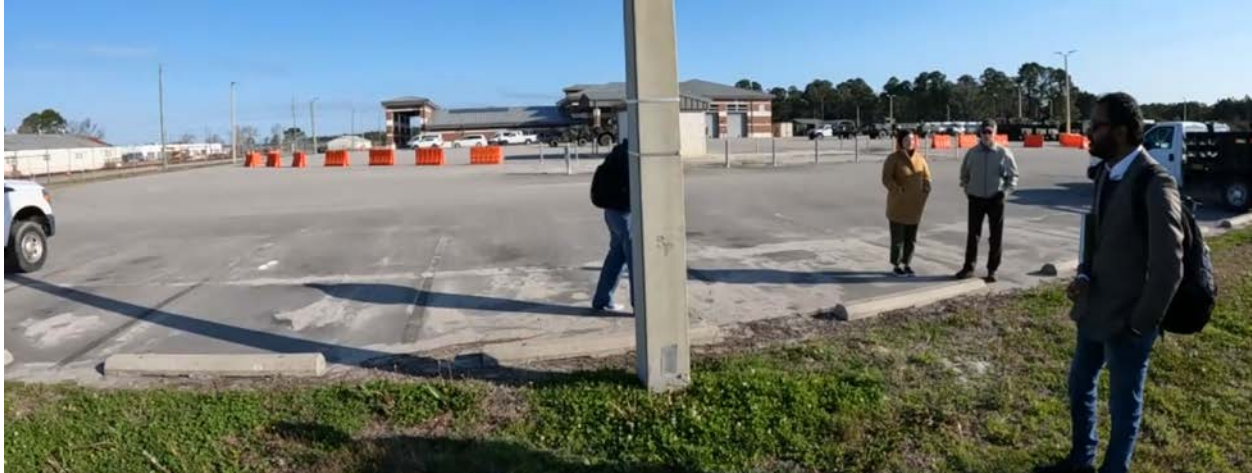
Figure 28. Building 773 parking lot location for EVSE (Pole Number 73243-45015)
