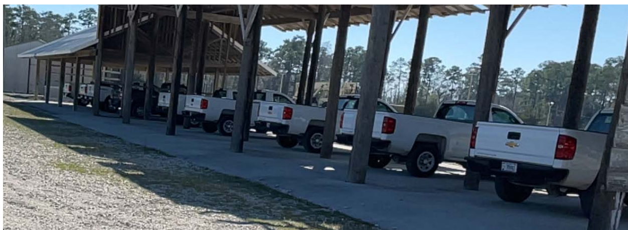
Figure 24. The backside of Lot 200 parking structure
