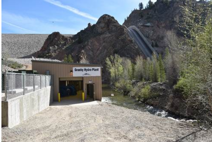
Figure 9. Granby Dam Hydroelectric Project – 1.2 MW. Photo courtesy of NWCD
