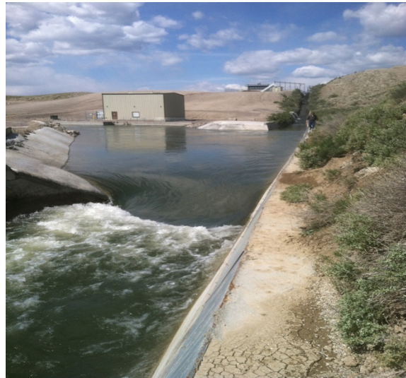
Figure 8. South Canal Drop 3 Hydroelectric Project – 3.5 MW. Photo courtesy of DMEA
