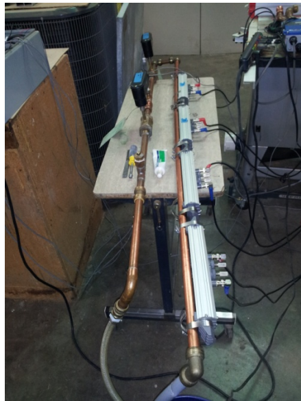
Calibration of four ultrasonic flow meters against turbine flow meters
