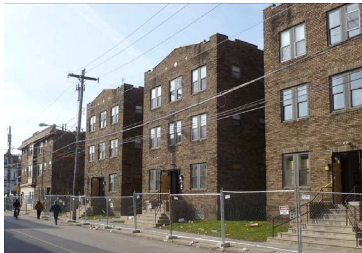
Figure 1. Street view of the 56 th and Walnut Street rehabilitation project
