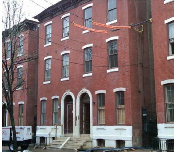
Figure 2. Street view of the Temple II North Gratz rehabilitation project
