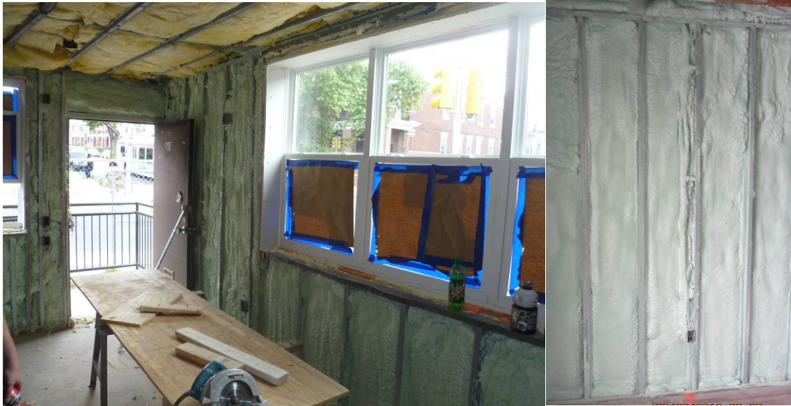
Figure 22. Above-grade wall insulation
