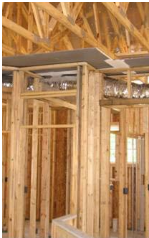
Figure 1. FDC after rough framing
