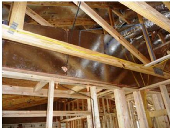
Figure 9. Radiant barrier backer board for standard batt insulation at knee wall installation
