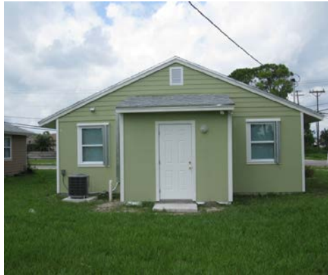
Figure 11. Completed exterior HPWH closet
