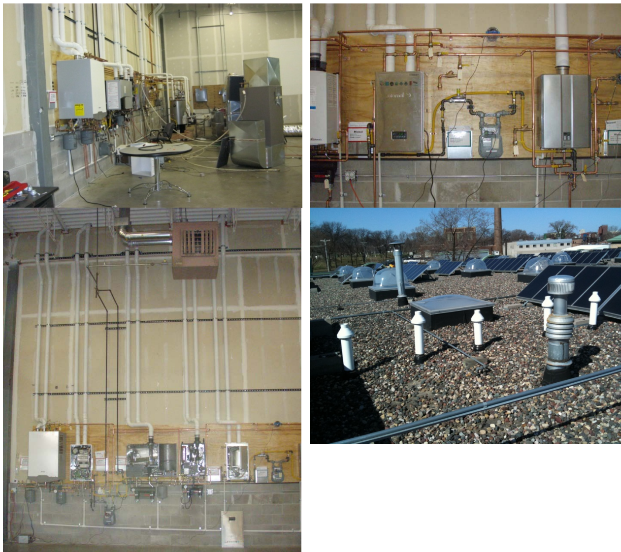
Figure 6. Photos of test laboratory with combi system installations and venting terminations
