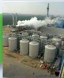
Biomass Conversion Technology
