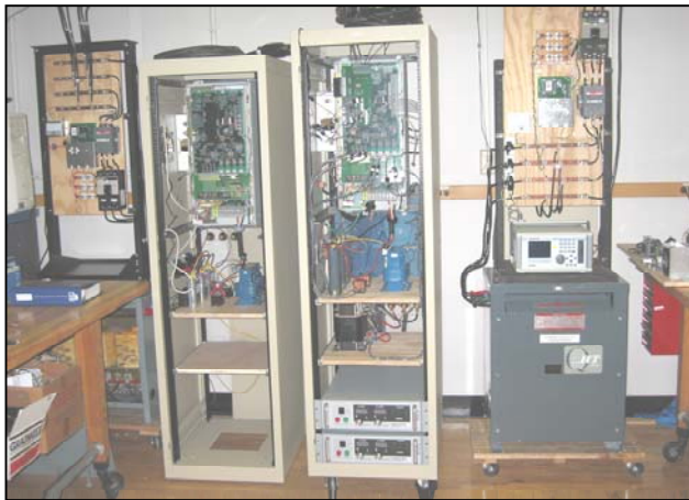
WisPERC's microgrid test hardware
