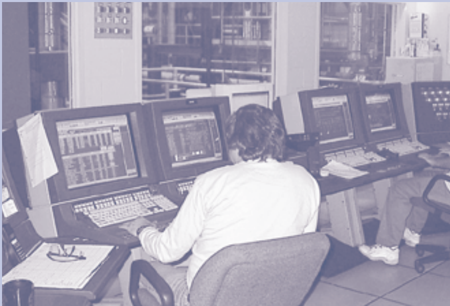
The AQC Optimizes Process Variables for Greater Energy Efficiency (Project 5)
